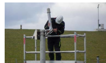
Installation of a probe on the 3 m. mast
